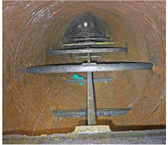
Robin Hood Shaft with haulage timberwork
